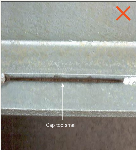
Figure 33: Overlapping Areas - Venting Unsatisfactory
